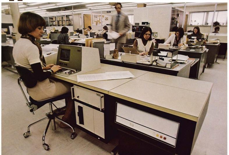
WCS/10 offers simplicity and economy based on the cost-efficient use of tape cassette storage. The system features a TV-like screen which guides the operator step by step. A typewriter-like keyboard with special-functions keys provides easy, push-button operation.
